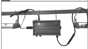
Mount remaining luminaire(s) to be connected in daisy-chain string in accordance with light plan.
