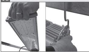
Supporting from below on either end, raise the LED module towards mounting structure and insert open hook of installed mounting bracket through the desired hole in the LED module end bracket.
